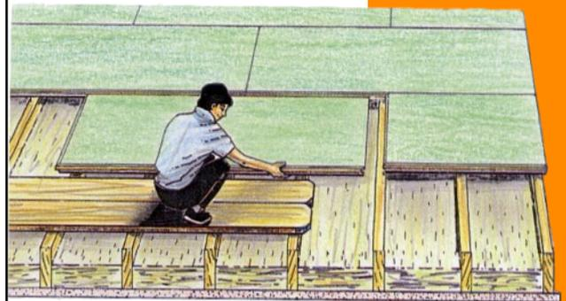
Additional Noggins will be required for unsupported ends of boards and edges at perimeter walls.
